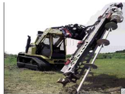
Installation of Screw Anchors
